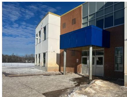
The playground doors at NFS.
